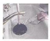
Hair can often clog a bathroom sink and potato peels and other food waste will plug up kitchen sinks. Regardless of the obstruction, unclogging both sinks is done the same way. Please use a screen on your drain for catching hair and anything else that does not belong in the drains. Do not use harsh chemicals, like
